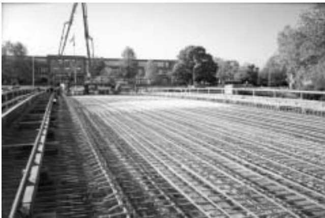
Fig. 2.4—FRP-reinforced deck constructed in Lima, Ohio (Pierce Street Bridge), in 1999.
